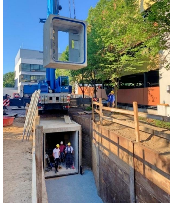
Figure 2.2 Pre-cast Multi-utility Tunnel Construction
